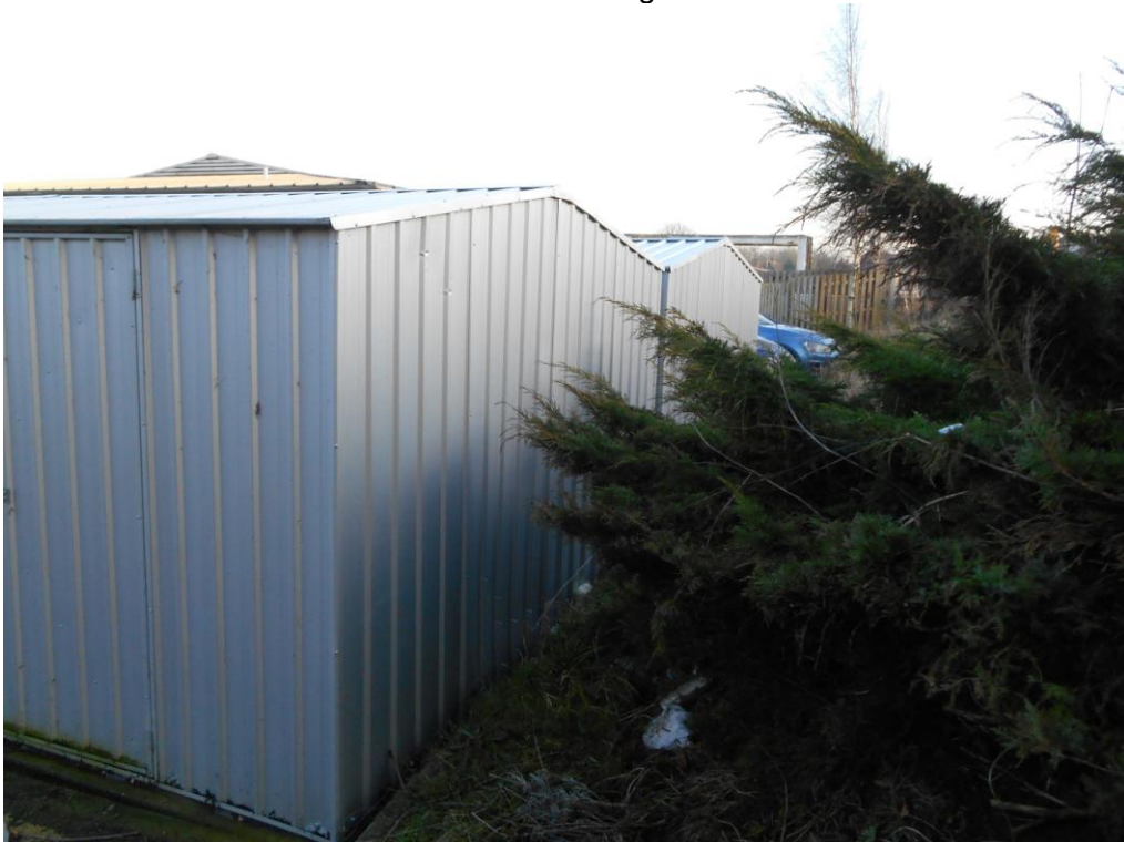
Rear of Garages
