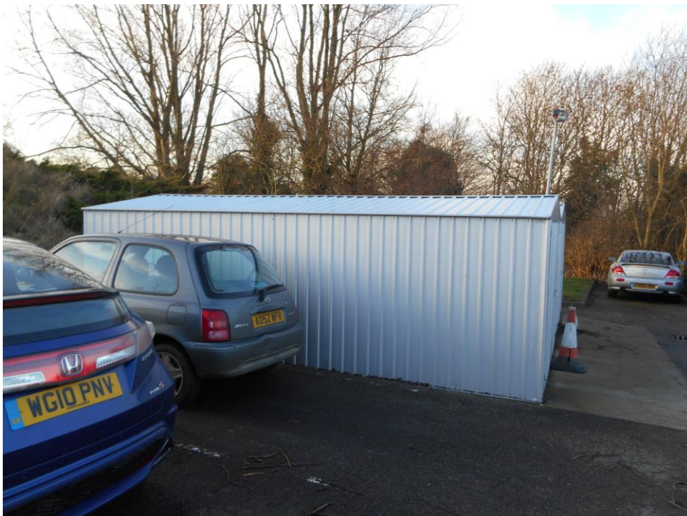
South Side of Garages
