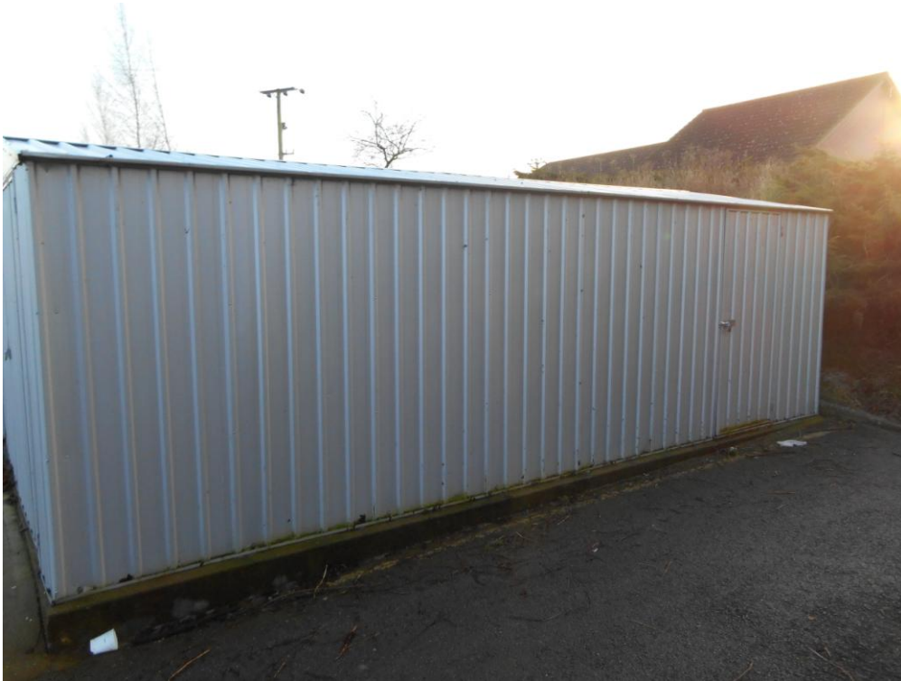
North side of Garages
